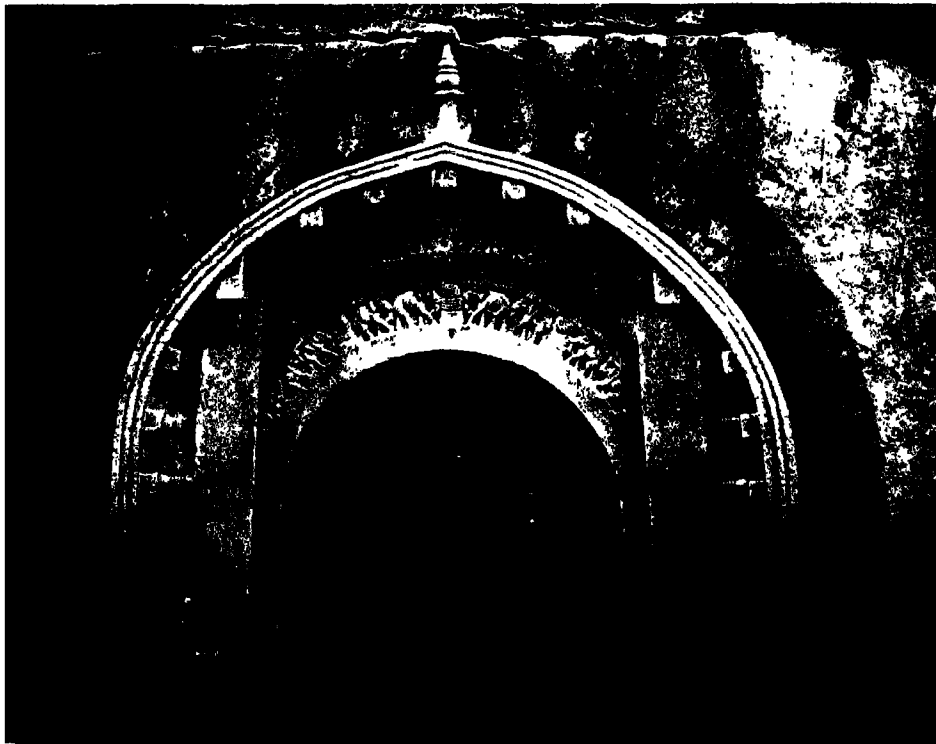
▲3b. Barābar Hills. Lomas Rishi Cave façade, 3rd century B.C.
